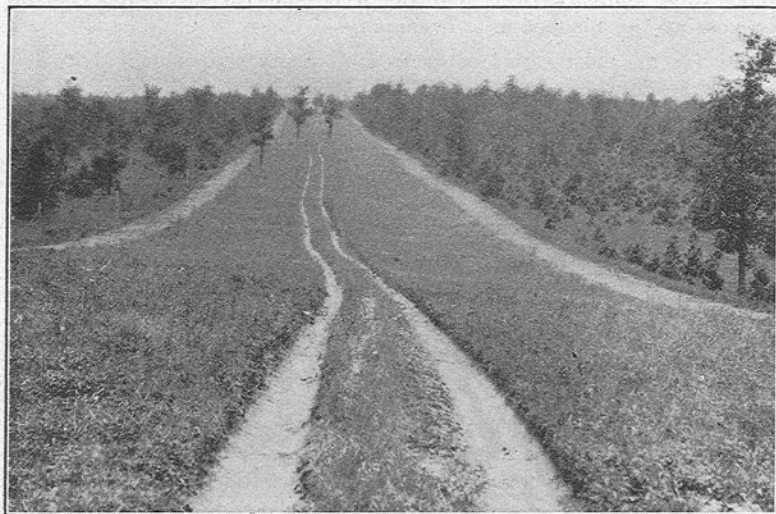
FIG. 20.—FIRE-LINE CONSTRUCTION ON PINE LANDS Double line type in the Huron National Forest.
