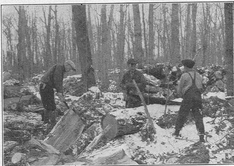
FIG. 4.—CUTTING CHEMICAL WOOD FROM THE TOPS AND CULL LOGS IN NORTHERN HARDWOOD OPERATIONS
