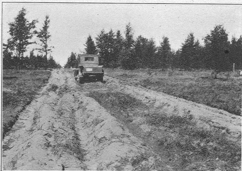
FIG. 21.—FIRE-LINE CONSTRUCTION ON PINE LANDS. Fire-line road on Michigan Fire Experiment Station.
