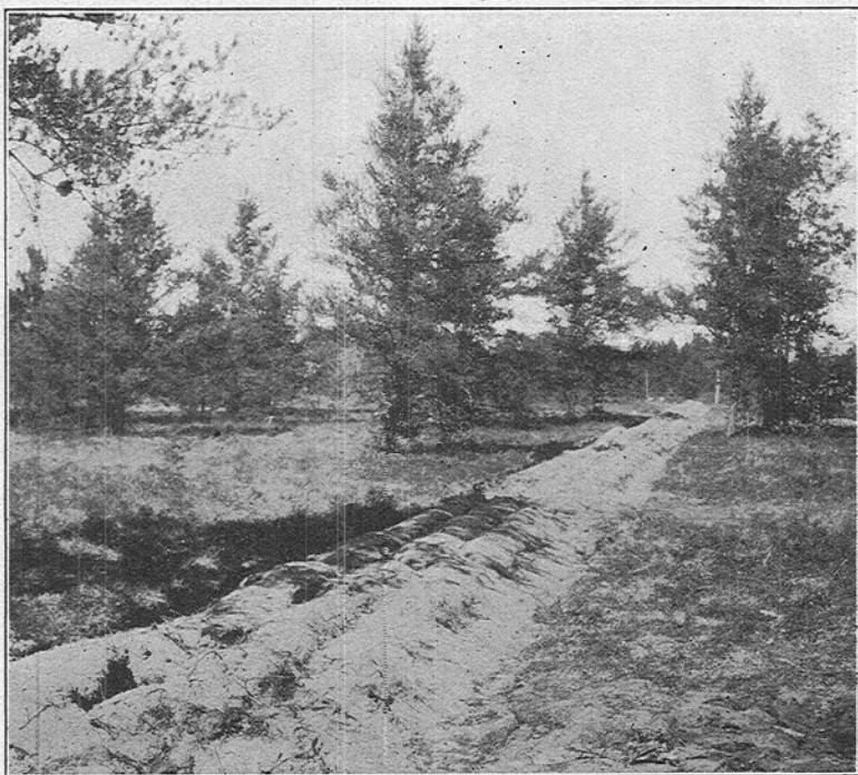
FIG. 22.—FIRE-LINE CONSTRUCTION ON PINE LANDS. An interior fire line at Michigan Fire Experiment Station.
