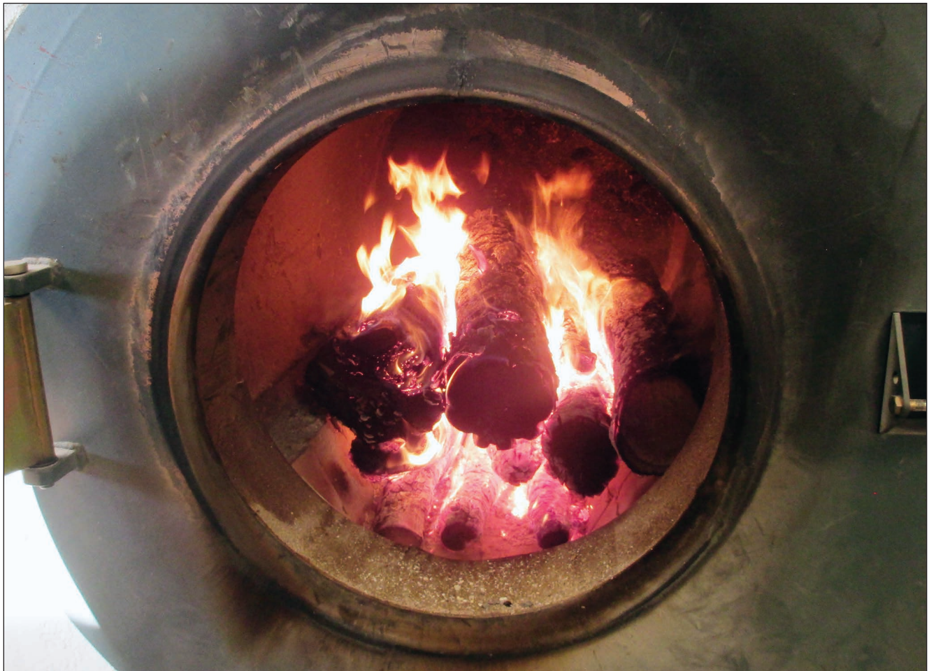
Figure 1—Many cordwood systems are designed to burn wood in an intense flame, quickly transferring heat to a water jacket surrounding the burn chamber. Note that in normal operation the door to the combustion chamber would be closed.
