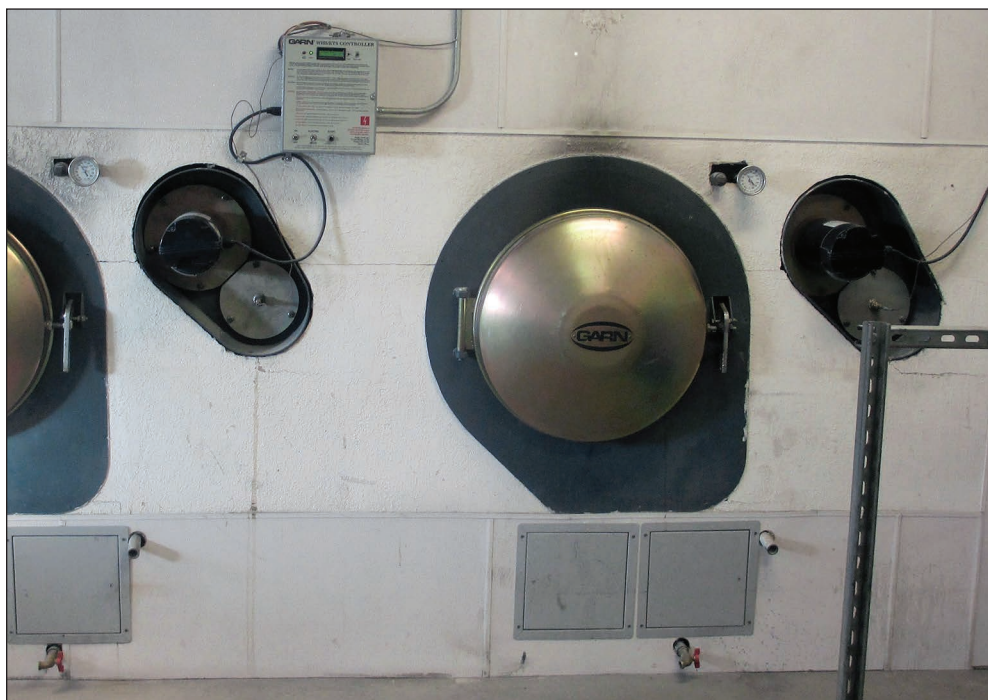
Figure 6—Front view of modular cordwood energy system, showing two independent units side by side (Gulkana Village Council, Gulkana, Alaska). Note that during normal operation the doors would be closed.
