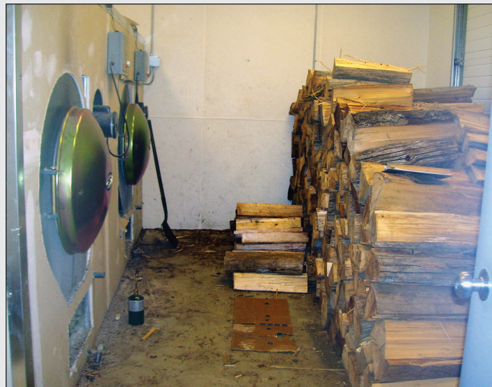
Figure 5—Fuel storage and loading area, Coffman Cove, Alaska. The final stages of wood drying take place in this room.
