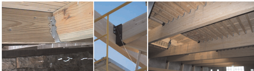
Figure 11 Typical joist hanger connectors.
