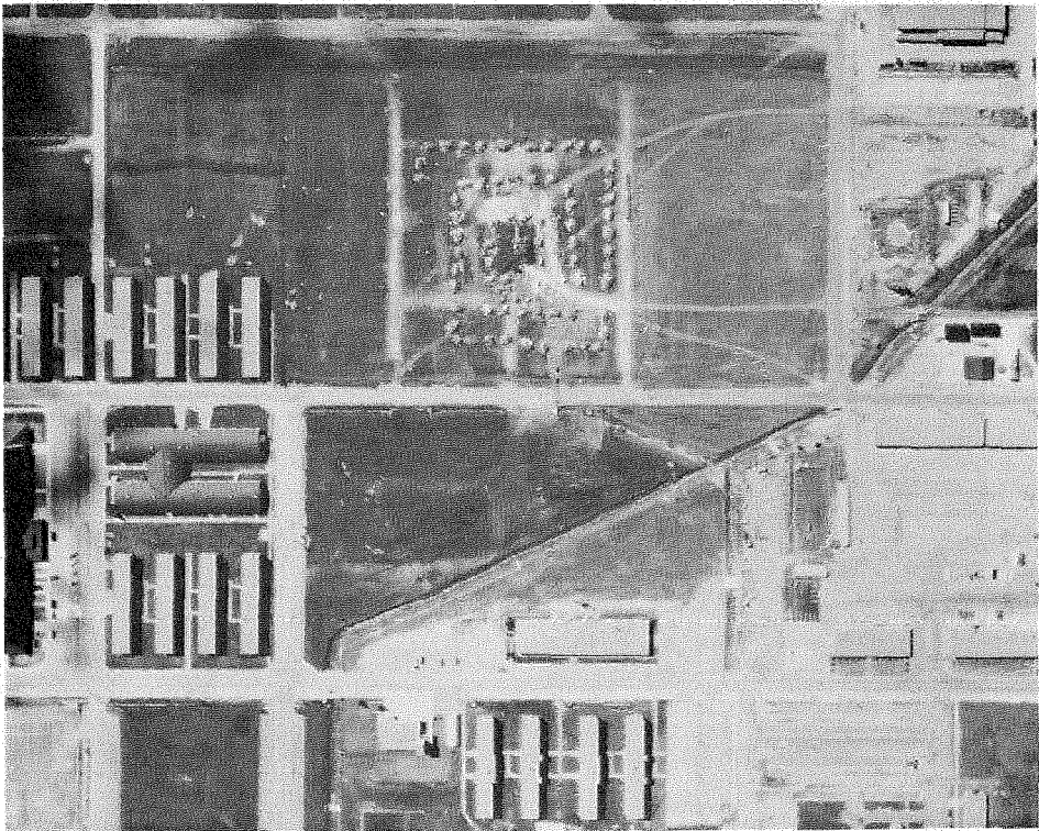
Figure 27.--Aerial view of Camp Parks Burn area.
