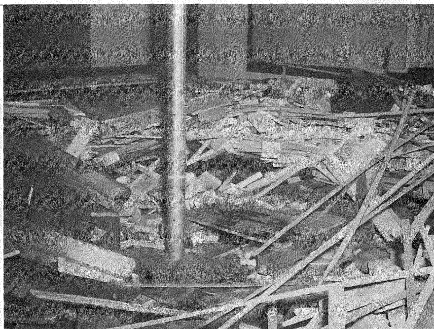
Figure 11.--Fuel distribution in classroom before Los Angeles Test No. 1.
