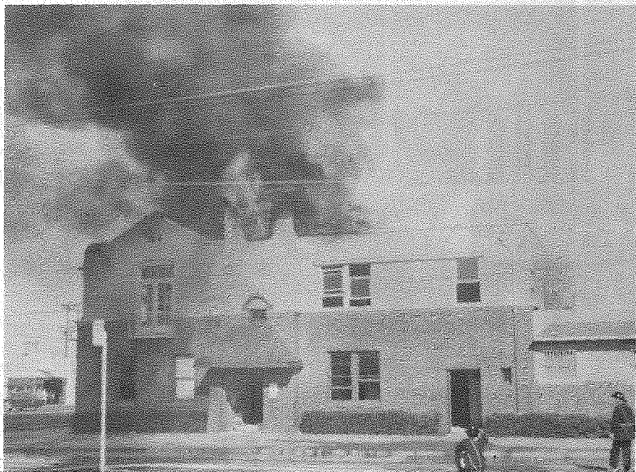
Figure 25.--El Cerrito municipal building shortly after ignition.
