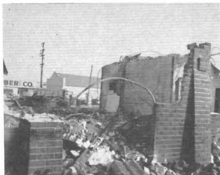
Figure 3. Rubble left after El Cerrito test.
