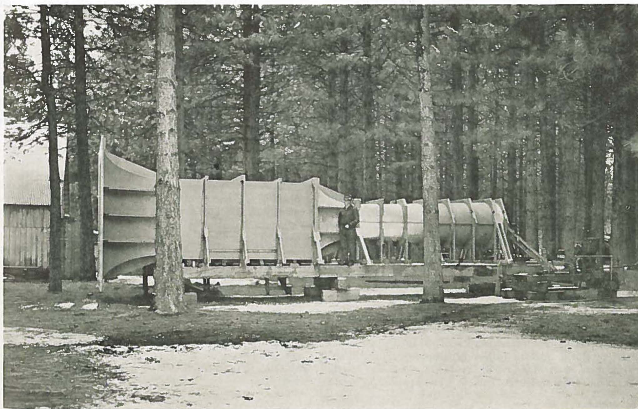
FIG. 15 WIND TUNNEL FOR FIRE-BEHAVIOR STUDIES
