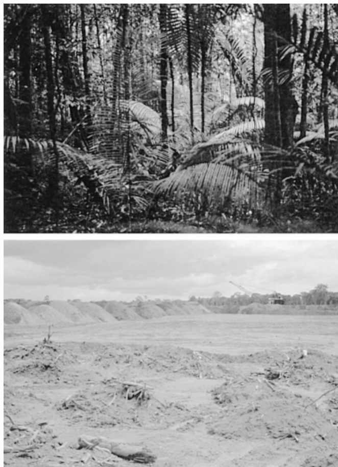
Figure 3. The Saracá plateau before and after bauxite ore extraction. Upper: Undisturbed primary forest; note abundance of palms in understory, typical of these forests. Lower: Site preparation, showing overburden hills (background, left) and topsoil and woody debris to be spread on site prior to planting (foreground).
