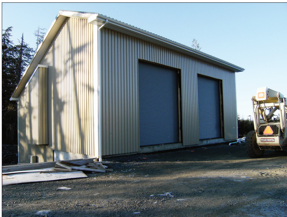
Figure 8—Front view of the Craig boiler building.
