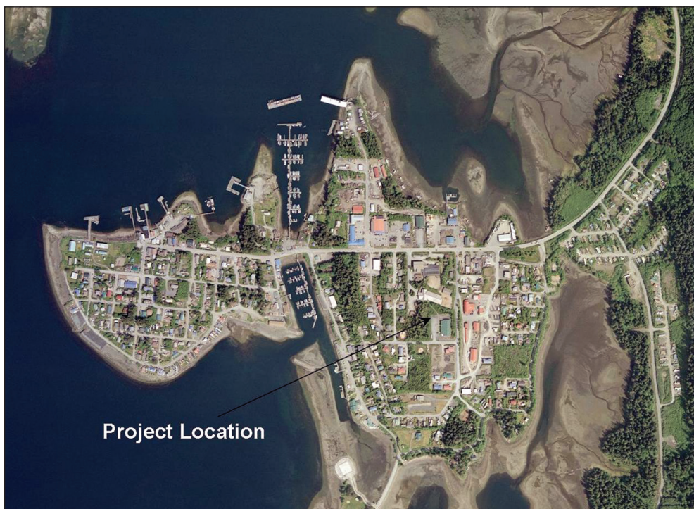
Figure 6—Location of the wood-fired boiler system, Craig, Alaska.
