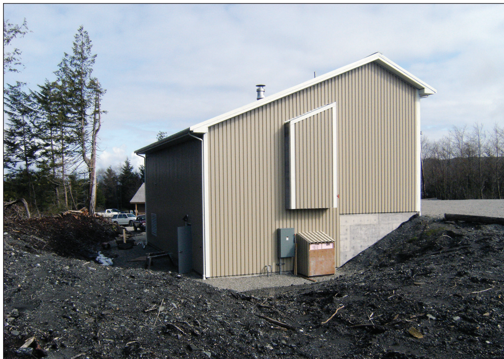
Figure 9—End view of the Craig boiler building.
