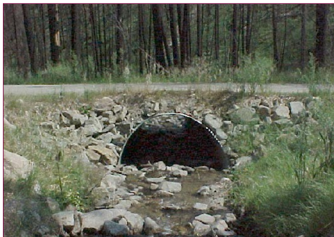
A new fish passage culvert on the burned area of the Bitterroot Forest.
