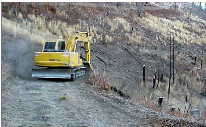
Excavator obliterating a road in the burned area of the Bitterroot Forest by reestablishing contours.
