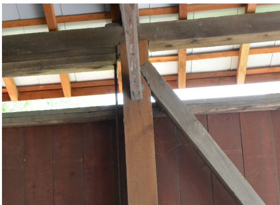
Figure 20: Simple angled bearing joints connection the diagonals t the vertical post for Eshlemann Bridge.
