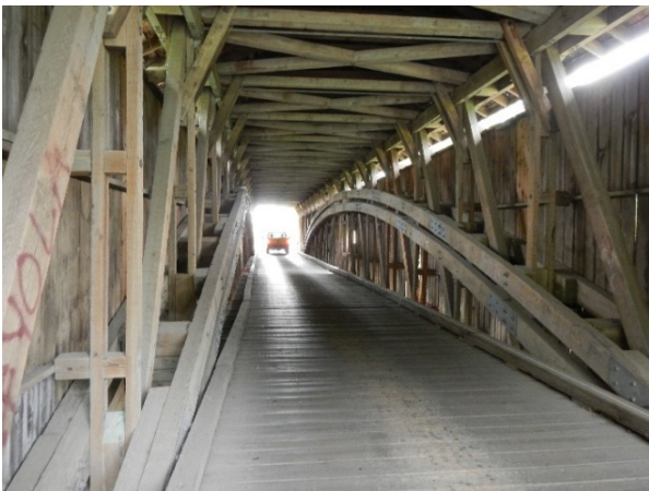
Figure 4: Interior view of Hunsecker Bridge
