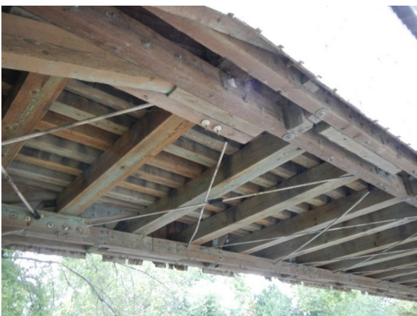
Figure 5: Floor System of Hunsecker Bridge
