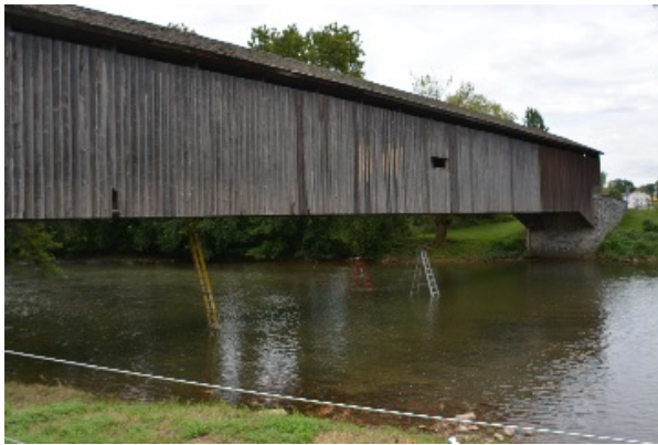
Figure 15: Global displacement measurements with transducers supported by aluminium ladders for Hunsecker Covered Bridge.
