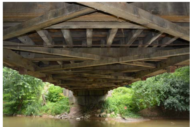
Figure 11: Floor System of Eshleman Bridge
