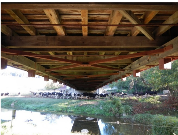
Figure 14: Floor System of Jackson Sawmill Bridge
