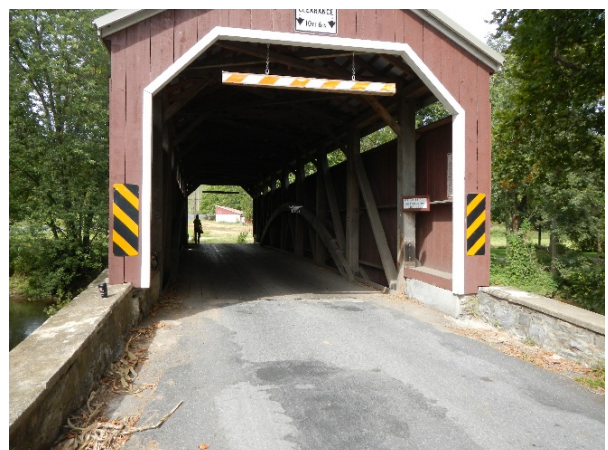
Figure 7: Interior view of Zooks Mill Bridge
