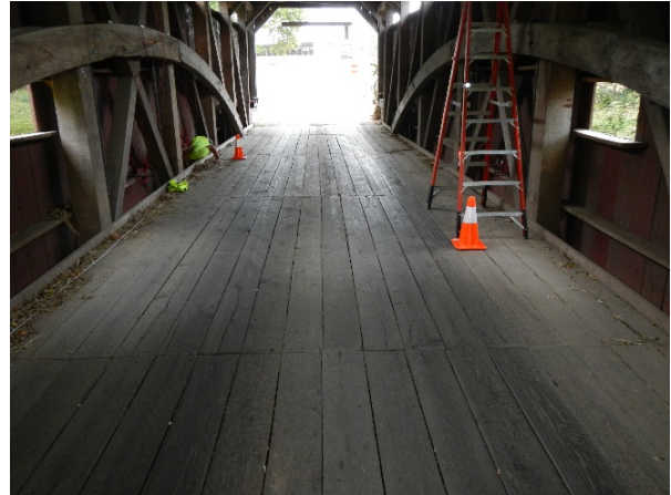
Figure 10: Interior view of Eshleman Bridge
