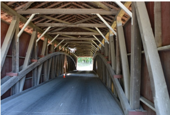
Figure 13: Interior view of Jackson Sawmill Bridge
