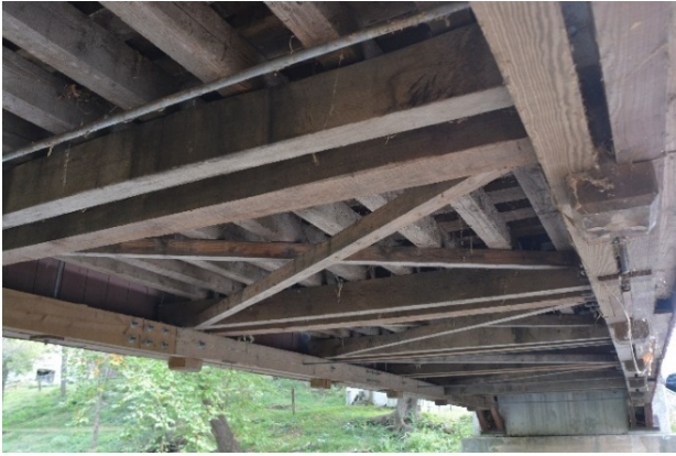
Figure 8: Floor System of Zooks Mill Bridge
