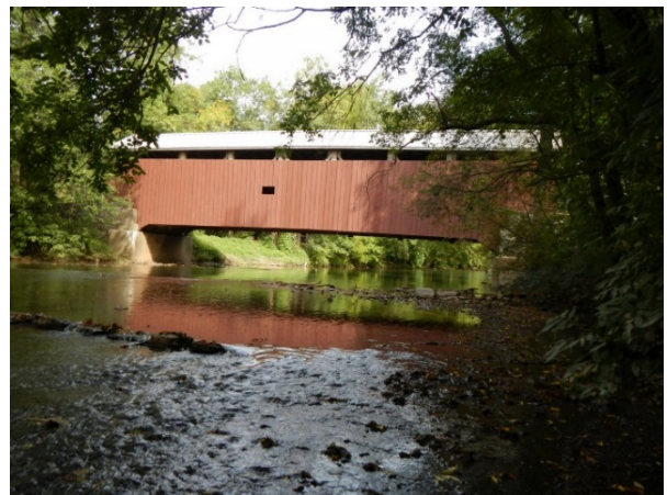
Figure 6: Profile view of Zooks Mill Bridge
