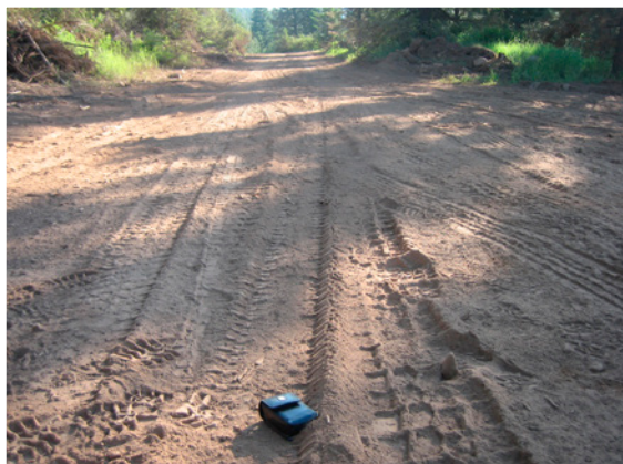
Highly disturbed soil with an increased risk of erosion on an access road to the site.
