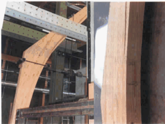
Figure 11: Failure of west arch at finger joint during third test
