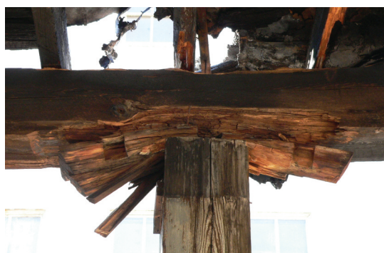
Fig. 1. Advanced decay of a timber girder and bearing plate. The deterioration was caused by years of exposure to roof leaks and resulted in the bearing plate being crushed. Photograph by Ronald W. Anthony.
