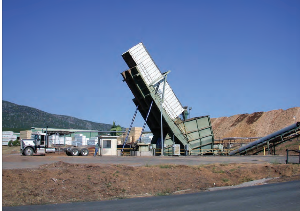
A woody biomass power generating facility in northern California.
