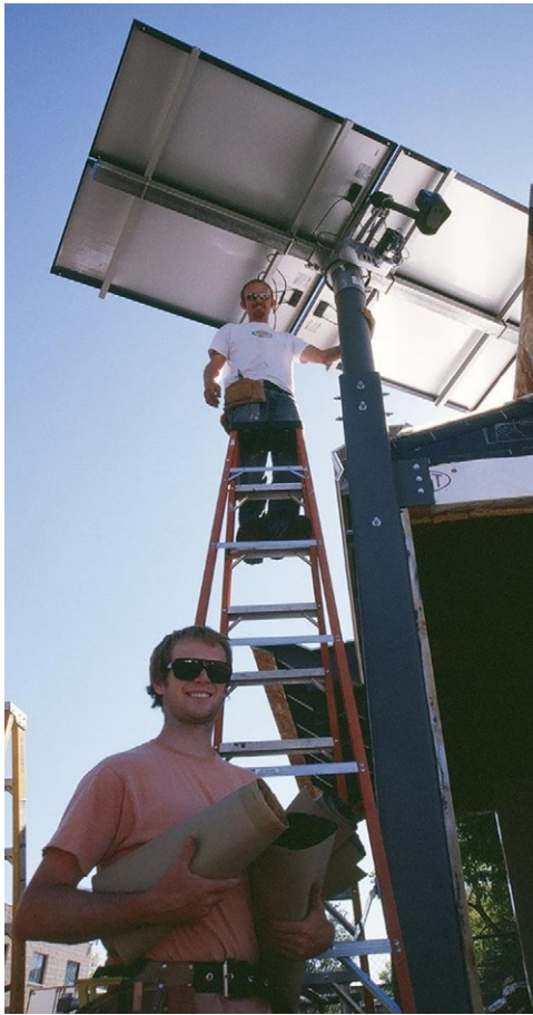
Figure 24. Student team members installing the dual-axis Sanyo 215 N photovoltaic (PV) solar tracker. The tracker rotates on two axes for maximum energy gains throughout the year and produces 142 kWh of electricity per month while helping power an adjacent commercial building.
