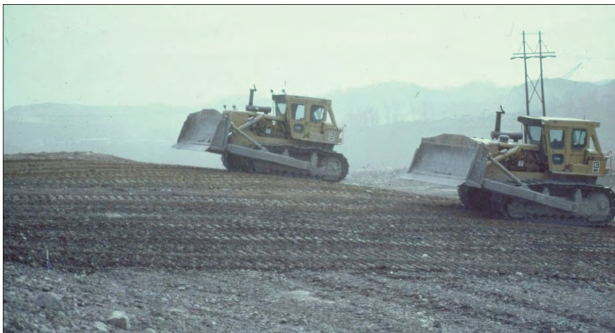
Figure 2-4.—Soil compaction due to heavy equipment operation on mine soils hinders survival and growth of planted trees. “Tracking-in” operations, such as those shown in the photo, are not recommended for mine sites on which trees will be planted, unless required to stabilize steep slopes. Photo by J. Burger, Virginia Tech, used with permission.
