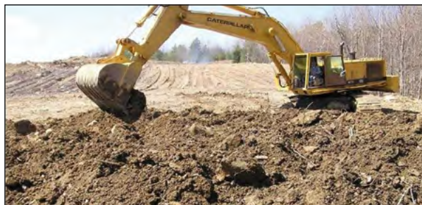
Figure 3-9.—Excavator leveling dumped topsoil piles. An excavator can be used to level soil piles without causing compaction and can be useful when the dumped soil piles contain stumps, logs, and other coarse woody debris. Photo by J. Burger, Virginia Tech, used with permission.
