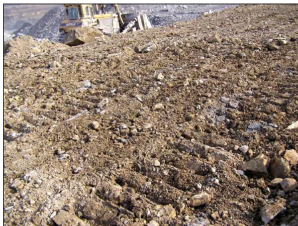
Figure 4-8.—A topsoil-substitute material that has been prepared for revegetation by using the low-compaction grading technique on a coal surface mine. The materials have been left in a loose condition. The rocky, rough surface will aid water infiltration and will not hinder the forest postmining land use that is being established on this site. Photo by J. Skousen, West Virginia University, used with permission.
