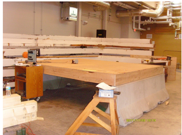
Figure 3—The laboratory-constructed wood floor system used for energy harvesting experiments.
