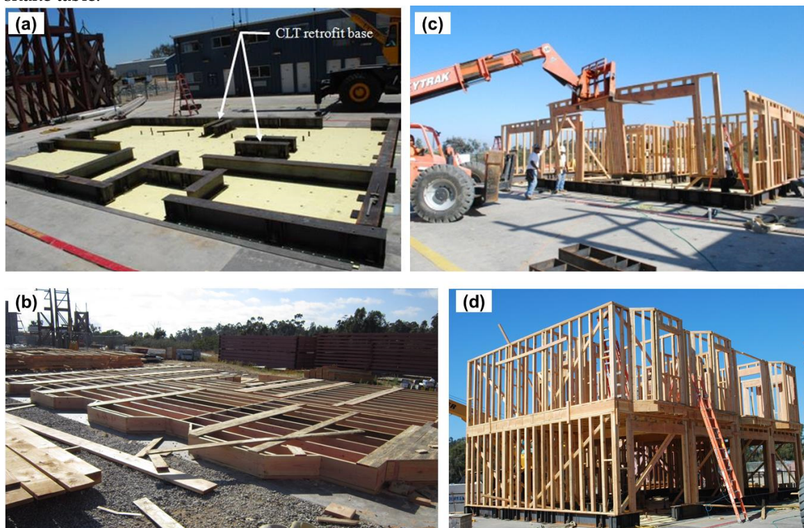
Figure 6. Construction of four-story building: (a) Installation of steel interface beams; (b) Prefabrication of floors and walls; (c) Erection of the first story with large openings; (d) Erection of the second story (stories 3 and 4 had the same floor plan as story 2).
