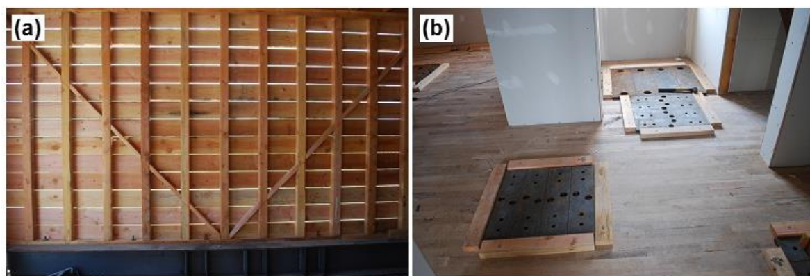
Figure 7. (a) Diagonal bracing at the west wall of the building at the first story; (b) steel plates attached to floor.
