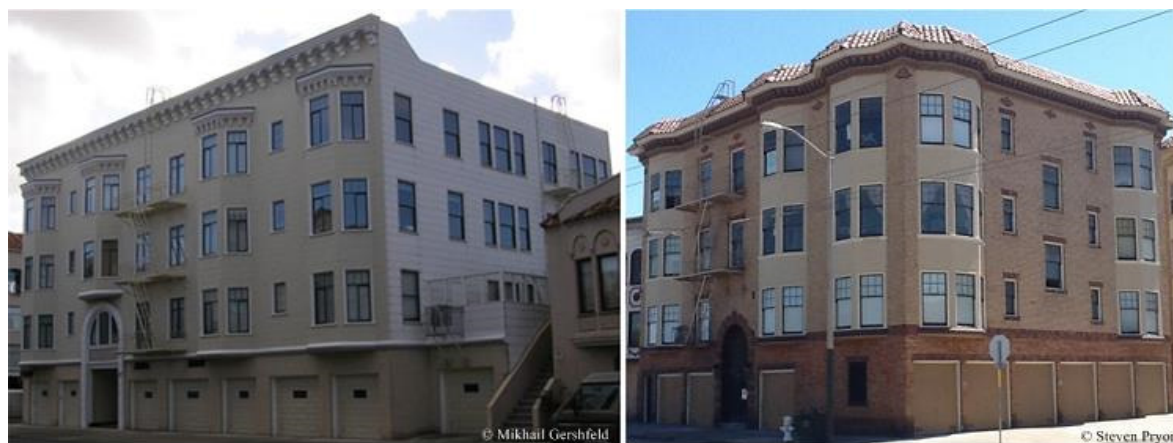
Figure 2. Soft-story wood buildings in the San Francisco Bay Area (Photos by Mikhail Gershfeld and Steven Pryor).
