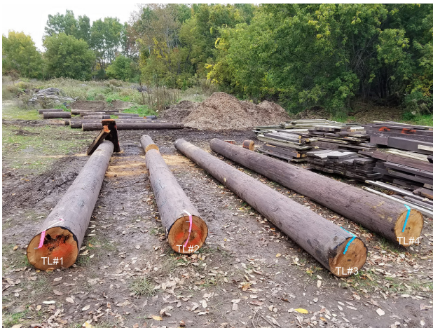
Figure 3. Sections from the four timbers that served as legs for the tower. Sections identified as TL#1 through TL#4 were the leg sections that rested on concrete support pads.
