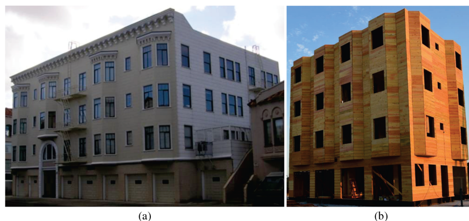
Fig. 1. Comparison of the architecture for (a) a soft-story wood building in the San Francisco Bay area (image by Mikhail Gershfeld); (b) the test building designed as part of the NEES-Soft project (image by Pouria Bahmani)
