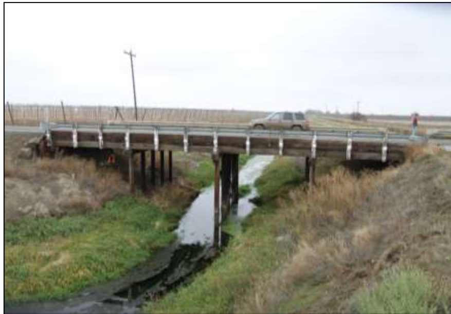
Figure 4: Durable example of a 75-year old sawn girder bridge located in Yakima County, Washington which still remains in satisfactory condition.
