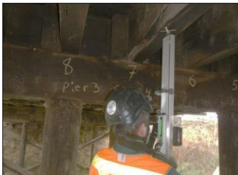
Figure 3: Resistance micro-drill, a minimally-invasive NDE tool, being utilized to inspect a sawn girder.
