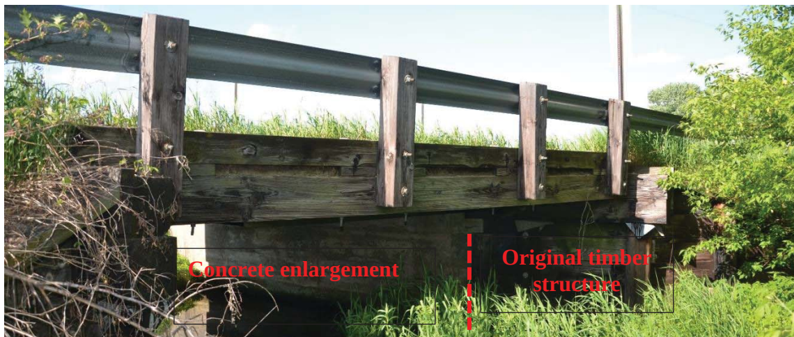
Fig. 4 Timber bridge enlarged with concrete members that has been wrongly codified as a TCC bridge
