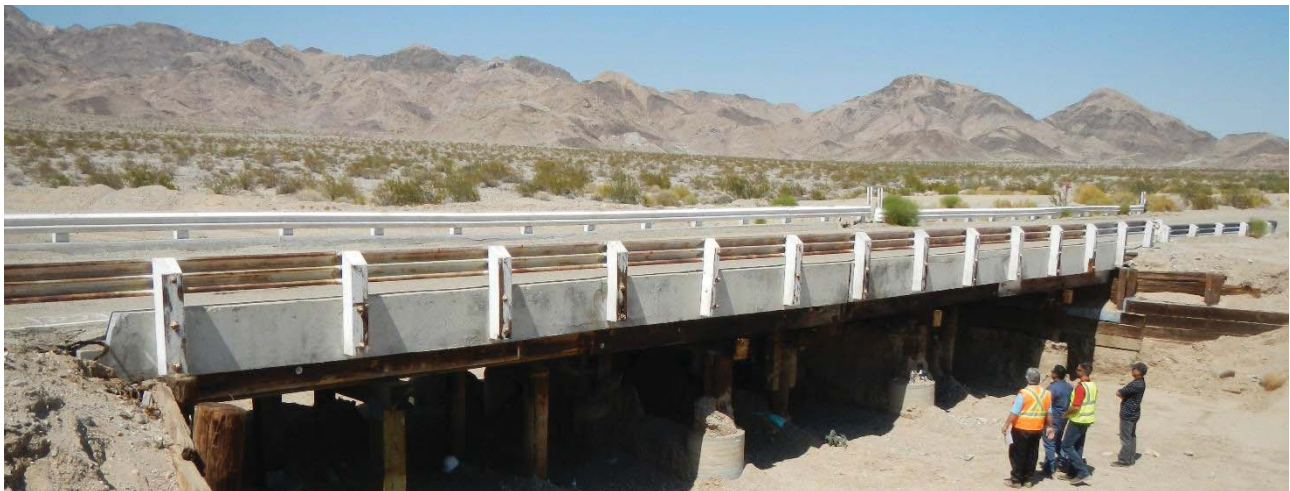
Fig. 3 TCC bridge along US Route 66 in California
