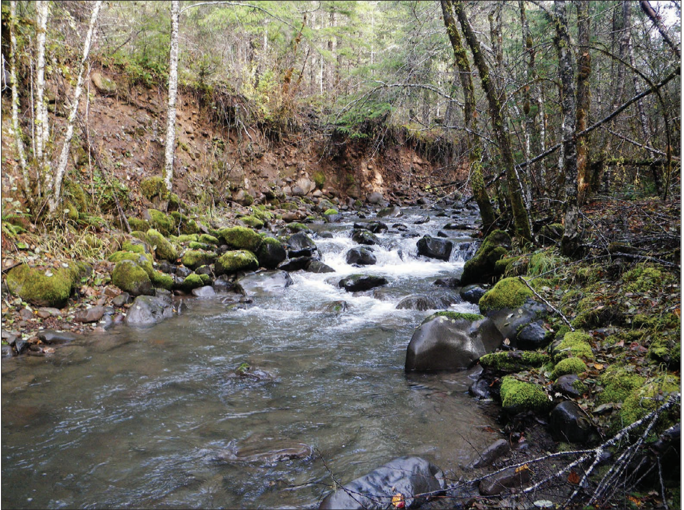
An example of stream bank erosion.
