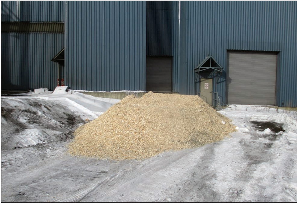
Figure 8—Outdoor wood storage of aspen chips at Aurora Power Plant.
