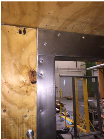
Figure 13. 14-gauge steel angles used to reinforce door frame.
