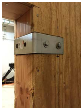
Figure 6. Simpson HL53 angle bracket used to reinforce the cane bolt latches.
