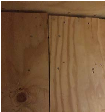
Figure 18. Interior damage caused by impact test of head jamb.
