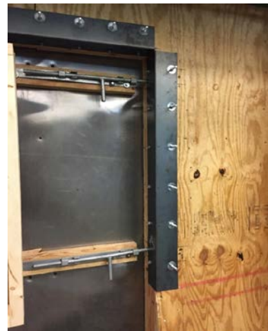
Figure 15. 14-gauge jamb reinforcement. Note use of both lag and through bolts to secure angle.
