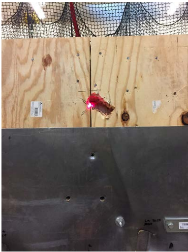
Figure 17. Exterior damage caused by impact test of roof-wall interface and head jamb.
