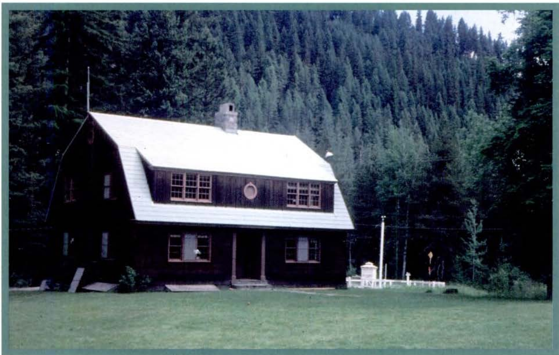
Headquarters building at Priest River Experimental Forest.
