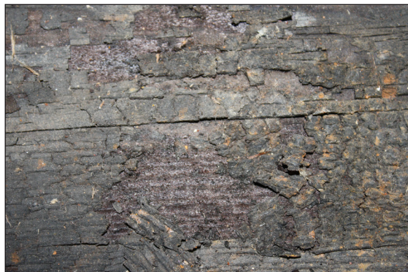
Figure 5. Brown rot decay on ceiling planking (side wall) of forward bilge.
