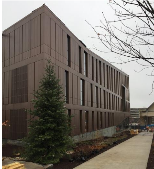
Figure 2: North exterior, along campus path
