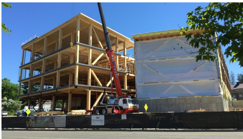
Figure 5: The building under construction
