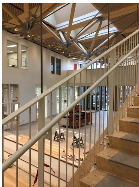
Figure 4: Commons under construction
