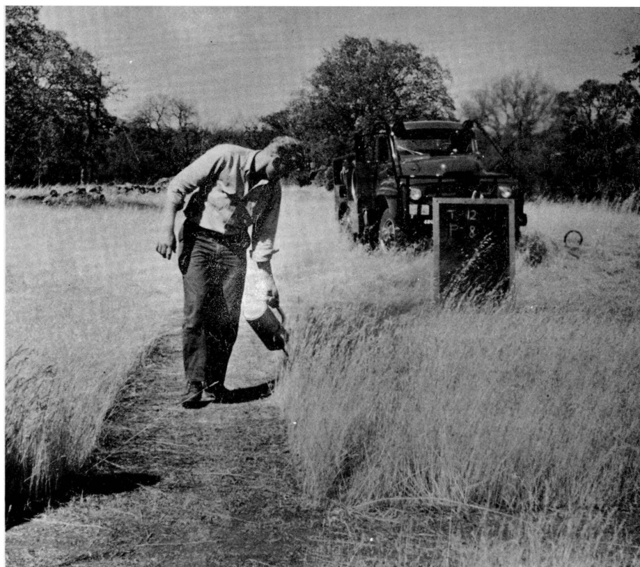
Figure 3.--Igniting a grass plot to evaluate the retardant characteristics of viscous water.
