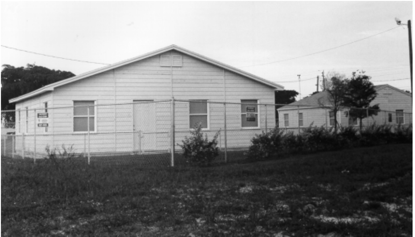
Figure 1—Test building with overhang (foreground) and test building with gutters (background).
