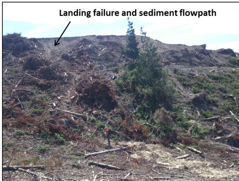
Figure 1 — Example of a sediment breakthrough to an ephemeral stream channel. This breakthrough resulted from a landing failure. (photo by Kristopher Brown)
