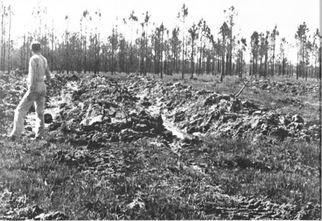
Figure 2.— High beds on intermediate site were elevated about 10 to 12 inches with a small dragline. Natural pines in background are stunted, and few will reach merchantable size.
