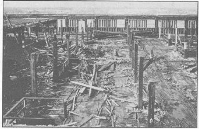
Figure 10—Demolition debris and construction waste represent a large untapped source of wood fiber.
