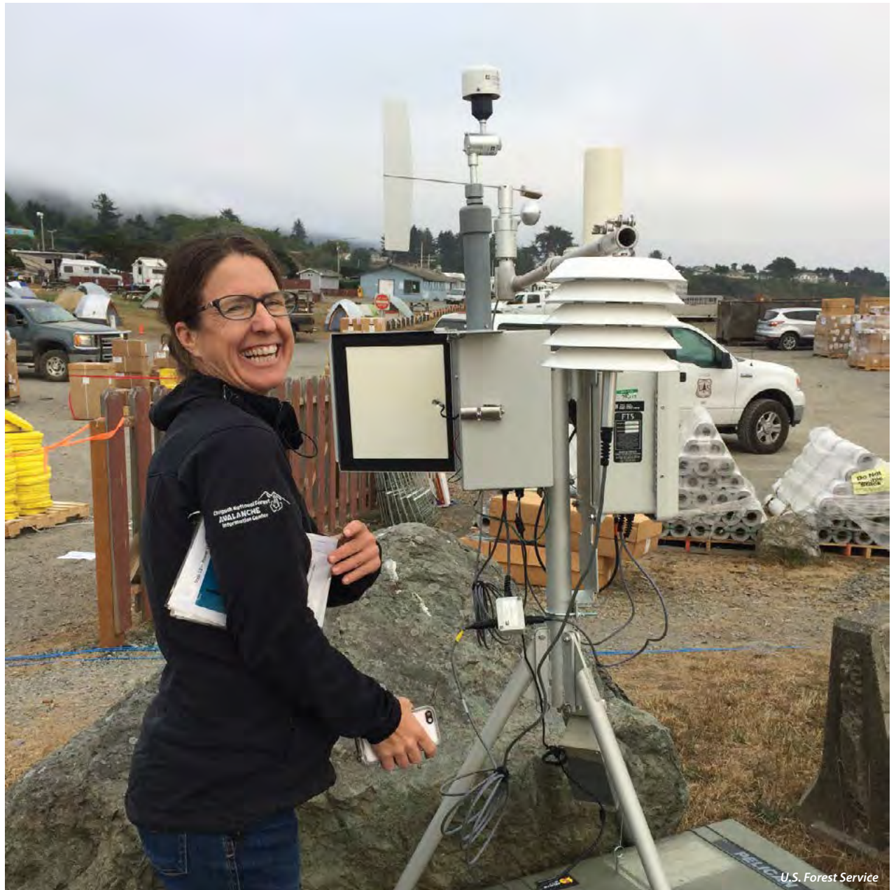
Air resource advisor Wendy Wagner sets up air monitoring equipment.
