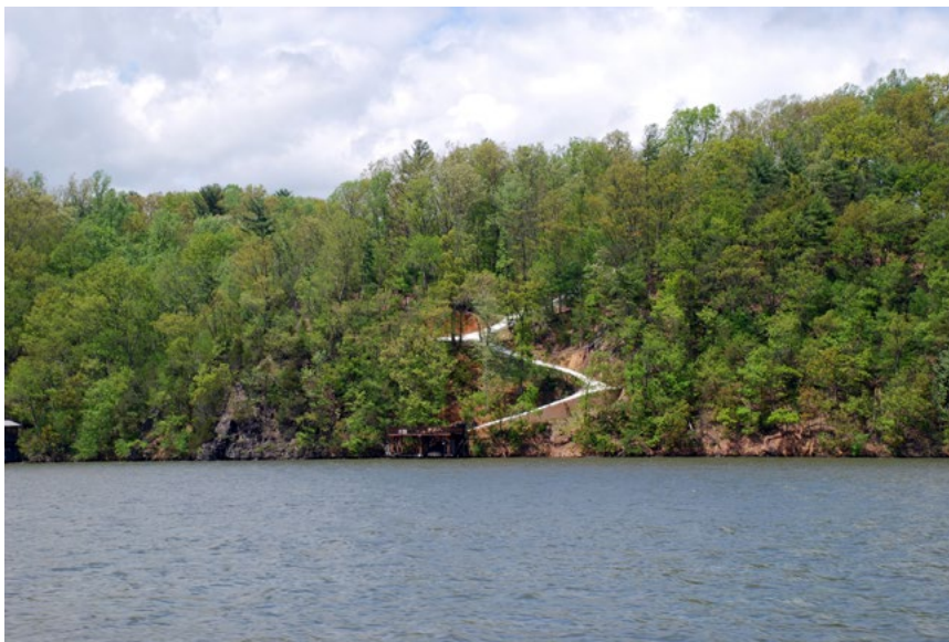
Figure 6.—Switchback access down to a boathouse on a steep shoreline detracts from scenic quality. It will be difficult to maintain and will continue to erode over time. Photo by P. Miller, used with permission.
