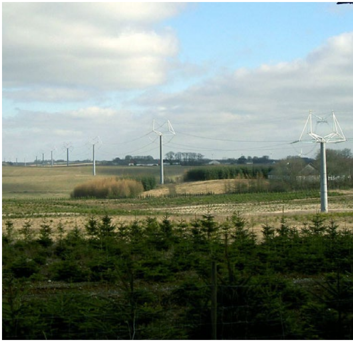
Figure 10.—The design pylon, the first pylon developed by the architectural firm Bystrup, is 60 percent the size of a traditional lattice tower. This design won a Danish government design competition in 2001. Referred to by local residents as “magic wands.” Photos by Bystrup Architects, used with permission.
