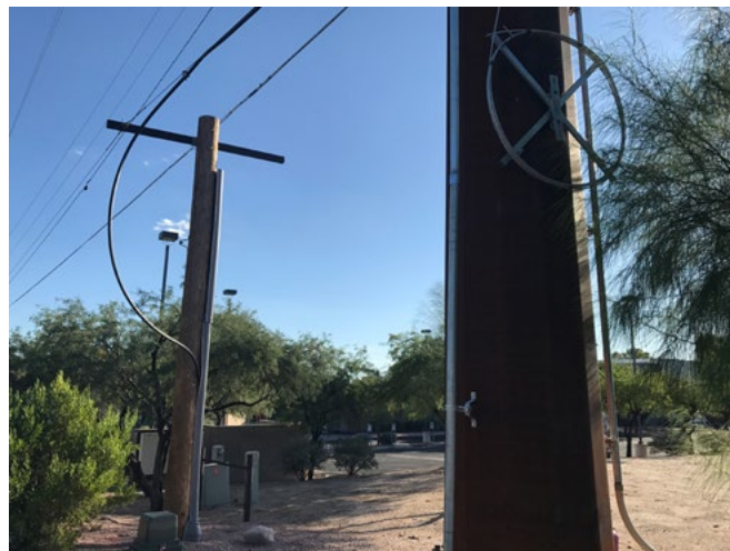
Figure 5.—Pole modifications, both by the original utility (leading to wires at top of pole [a]), and by tenants such as cable and communication carriers (leading to wires at bottom [b]), add to the visual clutter. Photos by Ellen Barth Alster, used with permission.
