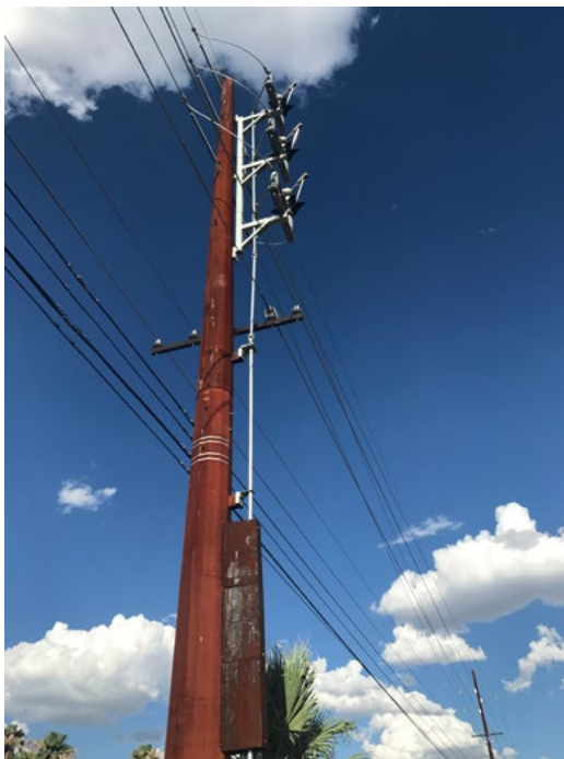
Figure 5.—Pole modifications, both by the original utility (leading to wires at top of pole [a]), and by tenants such as cable and communication carriers (leading to wires at bottom [b]), add to the visual clutter. Photos by Ellen Barth Alster, used with permission.
