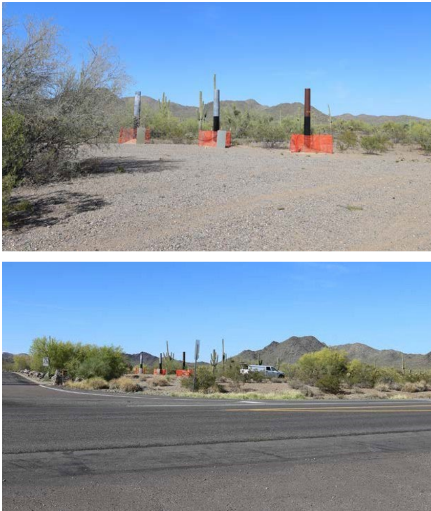
Figure 9.—Sample poles from Valmont for review by BLM. Photos by Brandon Colvin, U.S. Bureau of Land Management.
