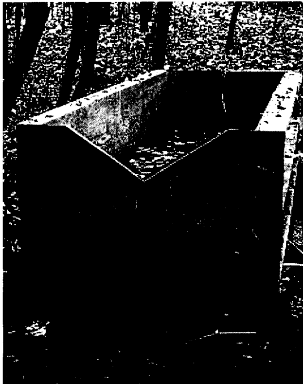
Figure 39.3. Photo – Monroe Street filtration box.
