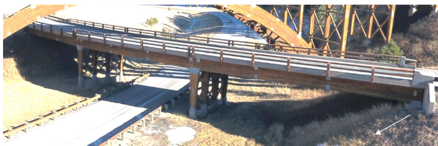
Fig. 2. Glulam timber girder bridge overview taken by the drone.
