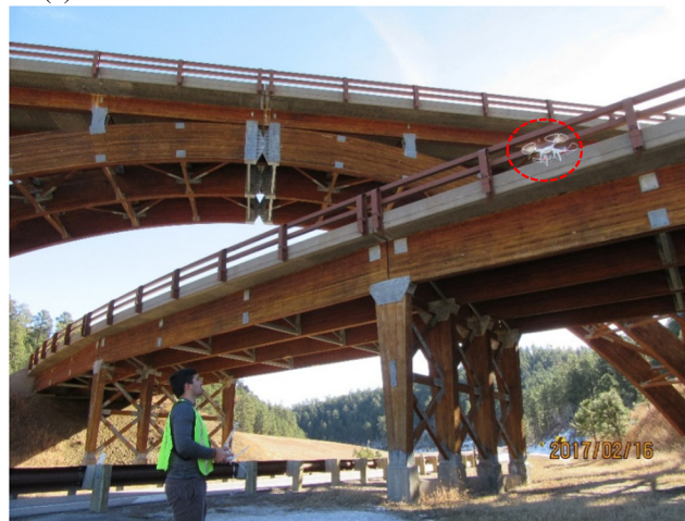
Fig. 7. Sample images obtained from the timber girder bridge inspection: (a) glulam girder bridge overview (taken by Junwon Seo using drone); (b) damage on timber girder bridge (taken by Luis Duque using drone); and (c) drone flying near girder (taken by Junwon Seo using digital camera).
