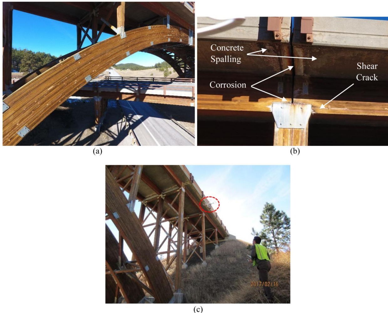
Fig. 4. Sample images for the drone-enabled bridge inspection: (a) close view of the arch; (b) identified damage on deck joint; and (c) operation of the drone near the bridge – Courtesy of Junwon Seo.
