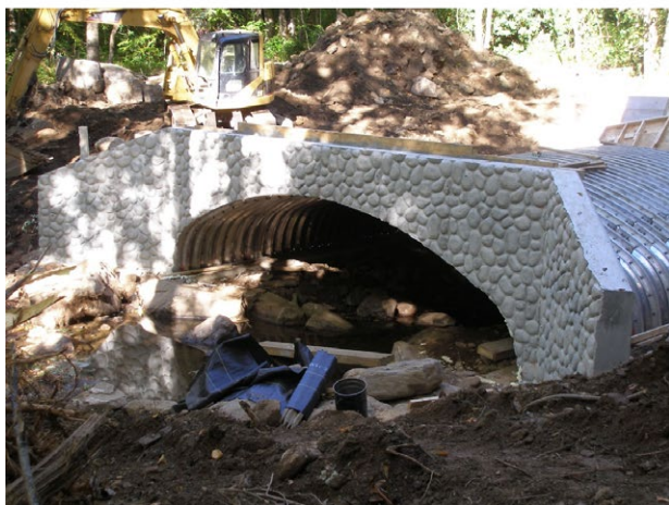
Figure 7. A partnership between Trout Unlimited and the Pisgah National Forest, North Carolina, to replace an undersized culvert (upper panel) with a flood-resilient bridge (lower panel) restored aquatic connectivity on Revels Prong and socioeconomic benefits to the local community. Photo credits: Trout Unlimited.
