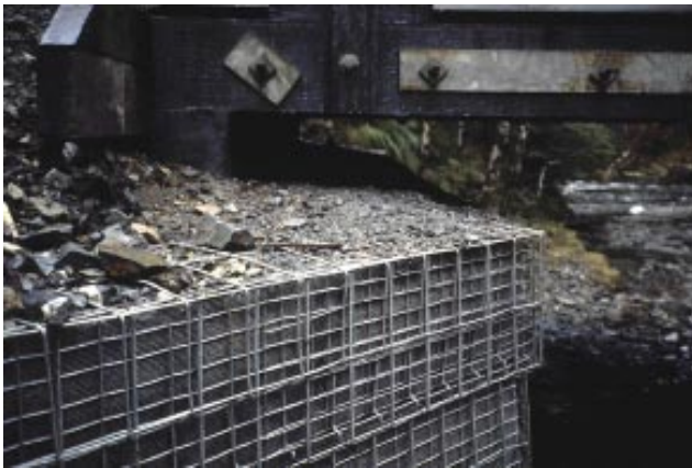
Figure 5—Welded wire basket abutments and timber sills.
