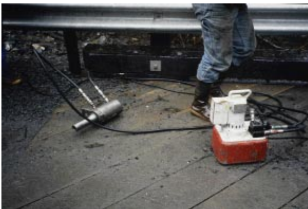
Figure 6—Hydraulic jack with built-in ratchet used for tensioning bars.
