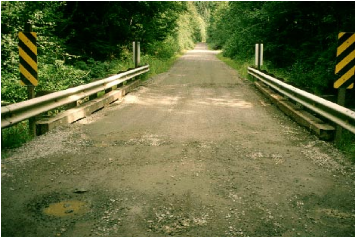
Figure 7—Completed Connell Lake bridge.
