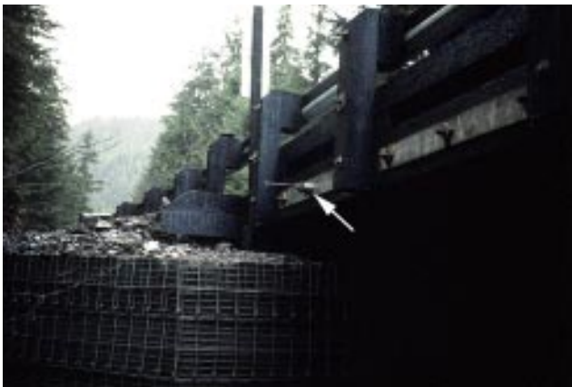
Figure 9—Load cell installed for measuring bar tension force.
