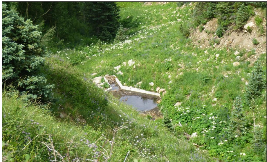
Figure 8 —This drain in North Creek Canyon is one of many diversions in the Abajo Mountains. Surface flows and riparian vegetation are absent below the drain (photo by D.M. Smith, USFS).
