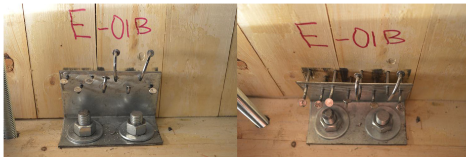
Fig. 9. Connector failure shear wall Test 05.
