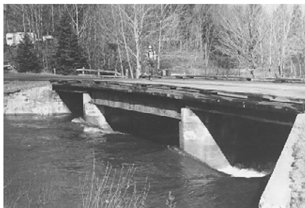
Figure 2—Big Erick's bridge prior to replacement (1980).
