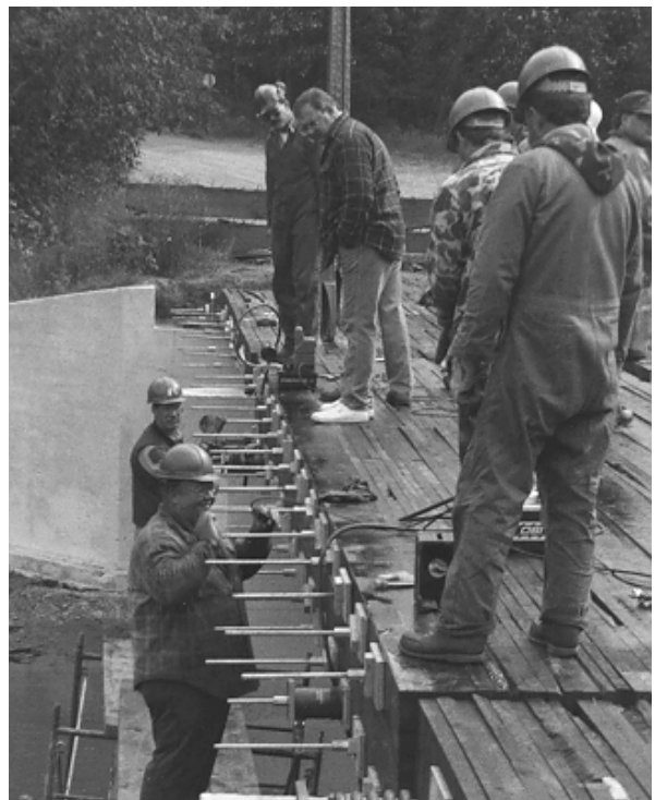
Figure 11—Two sets of deck stressing equipment were used to tension the stressing bars after deck placement.
