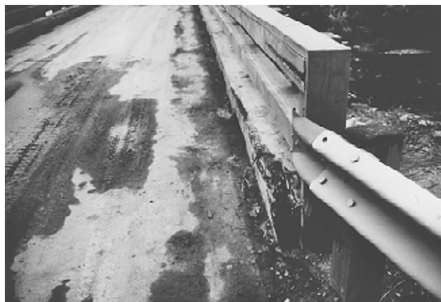
Figure 27—Vehicle damage to curb and rail system observed during a site visit near the end of the monitoring period.
