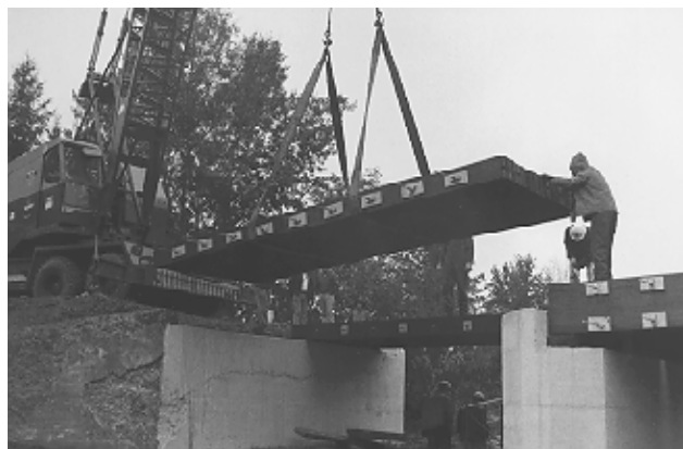
Figure 9—Placement of half-width panels with an overhead crane.
