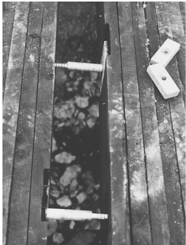
Figure 10—Connection between half-width panels was achieved by placing couplers on adjacent bars and stressing the entire deck together.
