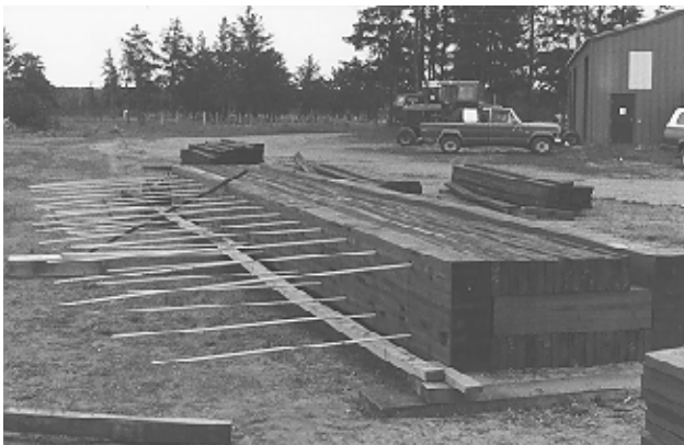
Figure 6—Prefabrication of the stress-laminated deck (top) and stress-laminated box (bottom) in half-width panels at an outdoor work site.
