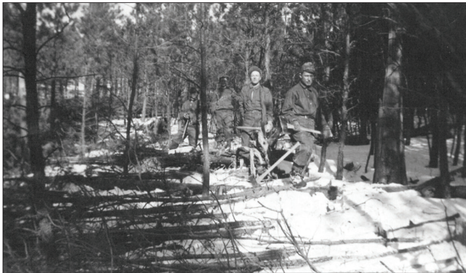
Figure 9 —For cutting the large saplings, the CC Corpsmen used double bitted axes and for small saplings they used brush-hooks, with much of the work accomplished during the winter (photo: Sanders 2004).
