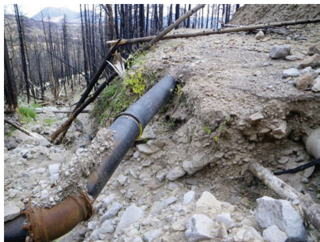
Fig. 17. Deep channel incision on the Waterline Road, Coconino National Forest, Arizona, after the 2010 Schultz Fire. Exposed pipe is part of the Flagstaff, Arizona, water supply system that was cut in 27 places by flood flows (Photo by D.G. Neary, USDA Forest Service).
