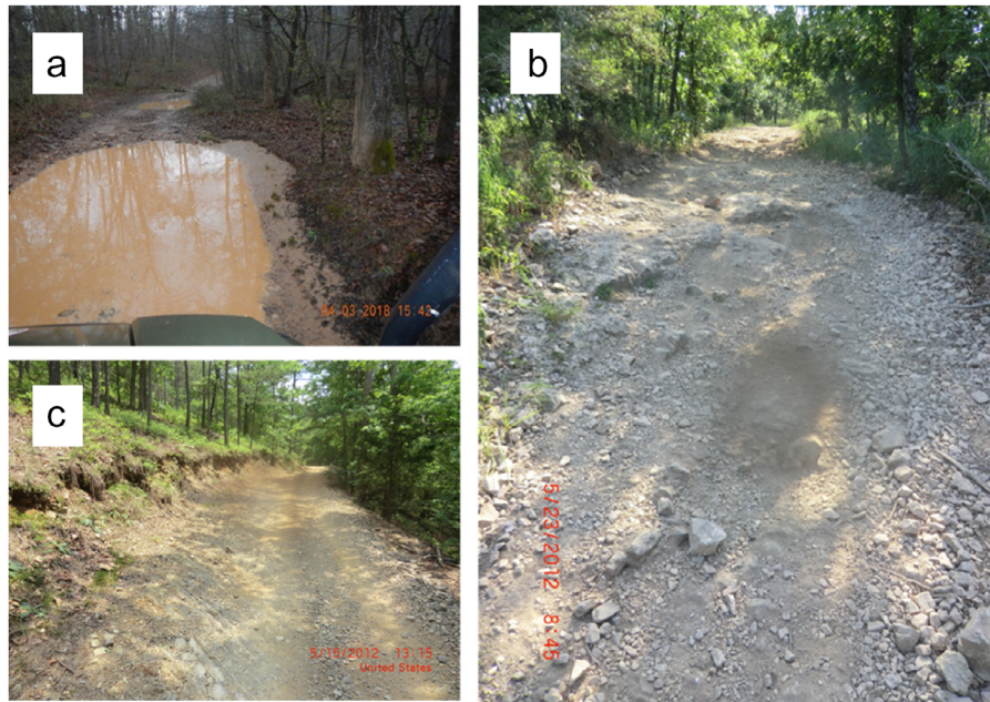
FIGURE 3. Examples of trail surface and sediment cover along WPG trails: (a) ponding and fine-sediment accumulation along low-gradient section; (b) bedrock outcrops and surface aggregate displacement along higher gradient section; and (c) rill formation and aggregate displacement along intermediate gradient section.
